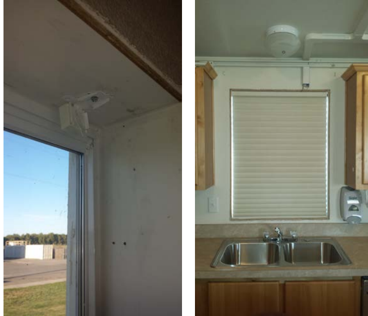
Figure 3.2. Mounting Bracket for the Cellular Shades (left) and Installed Hunter Douglas Cellular Shade (right)
