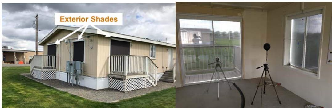
Figure 5. Exterior shades are installed in the PNNL Lab Homes. The exterior shades provide privacy and reduce glare, while allowing views during the day. (Photo at right shows view through the shades from inside the home).
