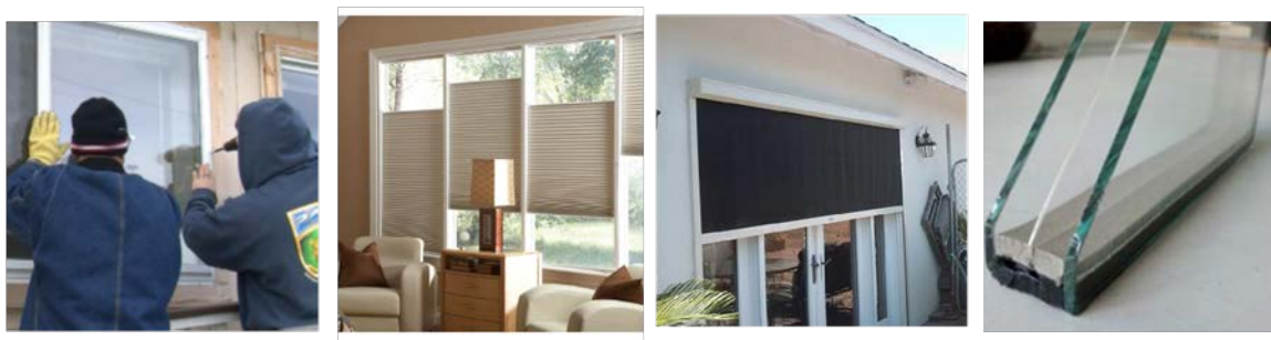
Figure 1. High Performance Window Technologies include (from left to right) exterior low-e storm windows, insulated cellular shades, exterior shades, and thin triple-pane IGUs. Sources: PNNL, AERC, and LBNL.
