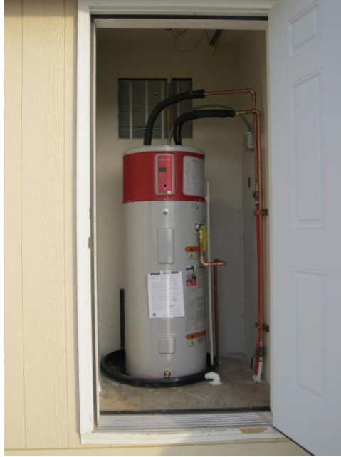
Figure 3.3. GE Gen-II GeoSpring HPWH Installed in Lab Home Water Heater Closet
