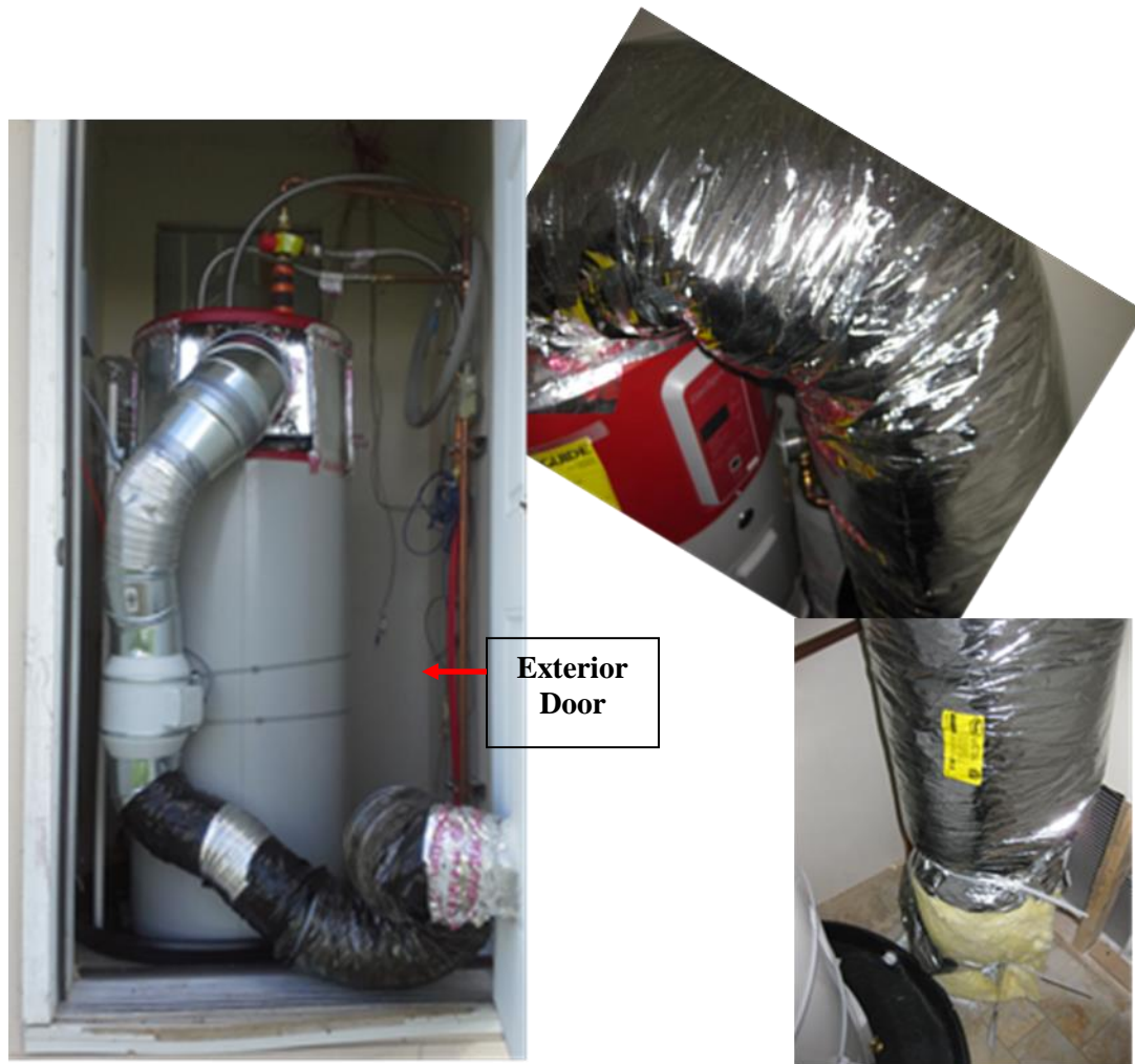
Figure 3.5. Left: Exhaust Ducting Approach on HPWH. Right: Supply Ducting Configuration on the HPWH
