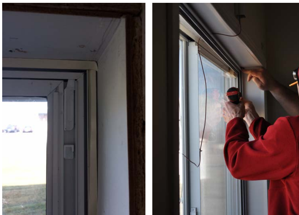
Figure 3.2. Interior Storm Window Weather Stripping and Installation
